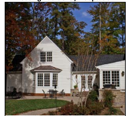
Housing Additions / Adaptation
