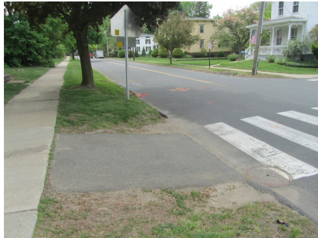
Figure 13: Hartford Avenue/Francis Street Crosswalk in Private Driveway
