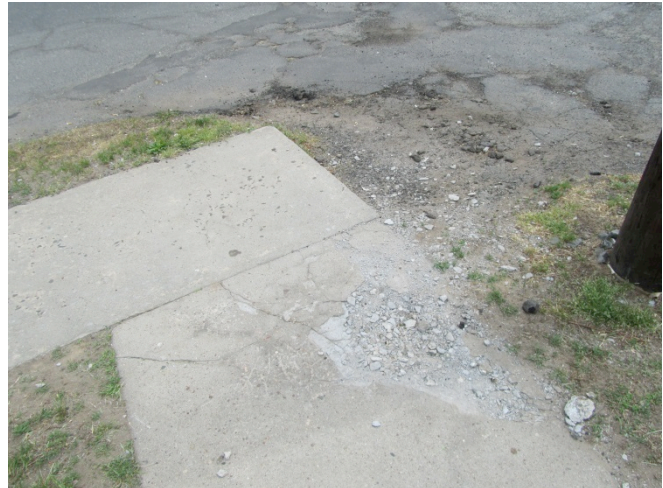
Figure 9: Hartford Ave/Avalon Place Broken Pavement at Handicap Ramp
