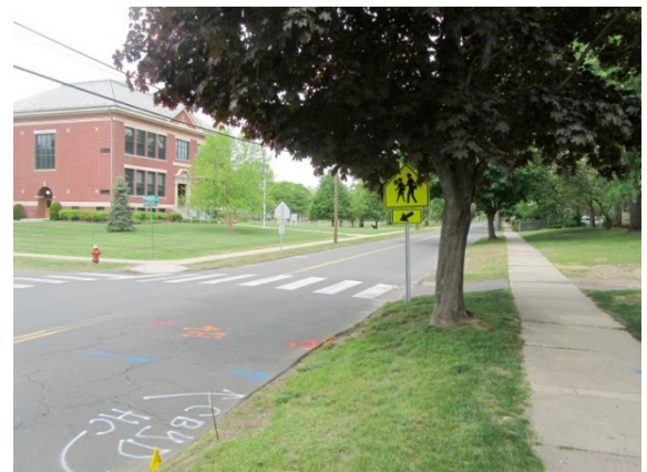
Figure 14: Vegetation Obscuring Visibility of SCHOOL CROSSING Sign on Hartford Avenue
