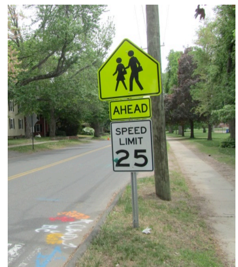
Figure 19: Newly Installed Signs Crowding Older Signs
