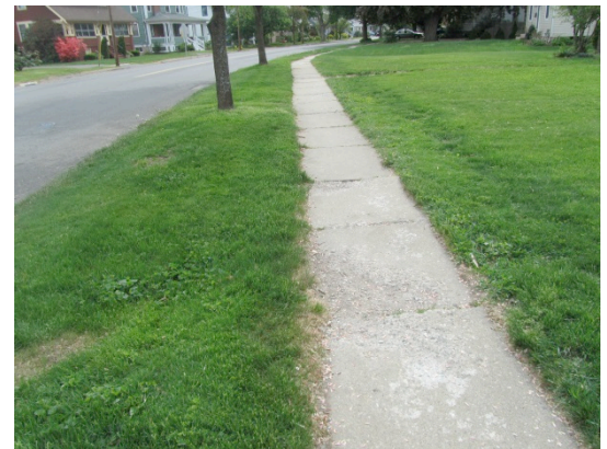
Figure 17: Church Street South Sidewalk Weathering
