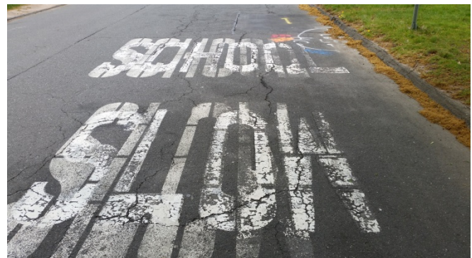
Figure 10: Poorly Painted SCHOOL SLOW Pavement Markings
