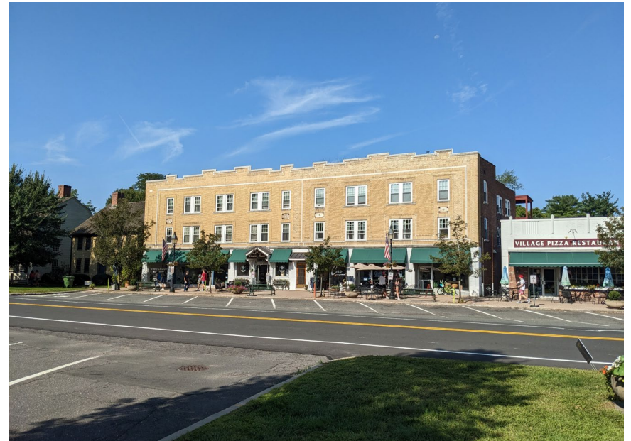
View of businesses on Main Street Source: FHI Studio
