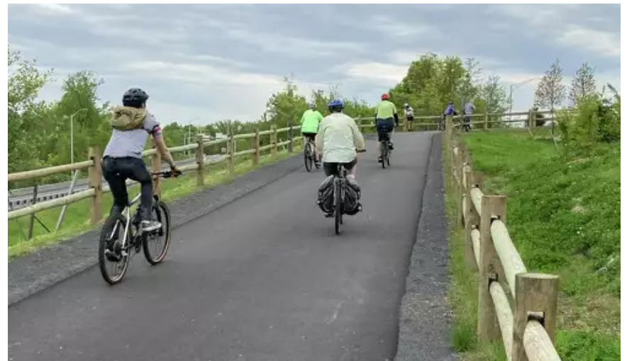
Wethersfield entrance to the Putnam Bridge Trail
