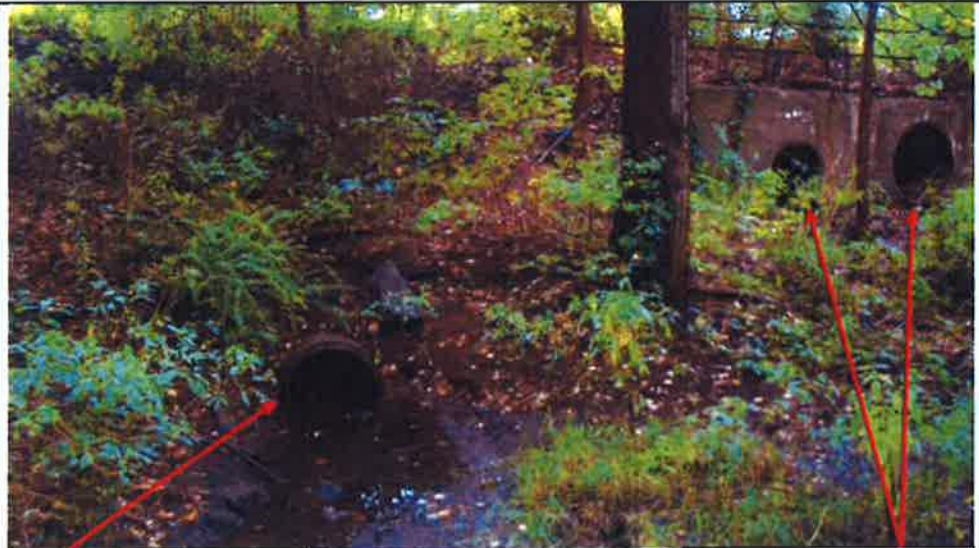
Auxiliary Spillway Outlet
