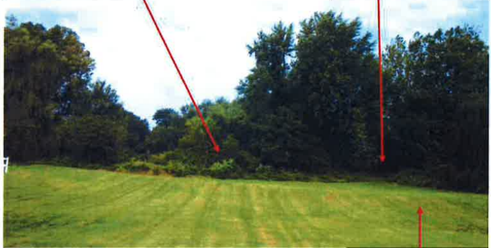
Auxiliary Spillway Dike
